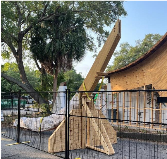
New Beam before putting it in place
