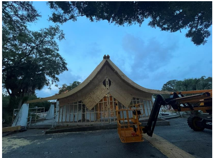
Both new beams in place
